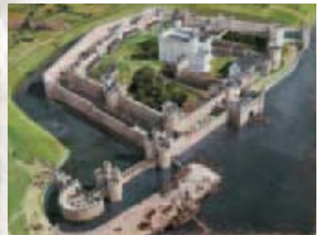
The outer curtain wall and the moat were both in place by 1300. It was now a concentric castle, because it had a double wall.
