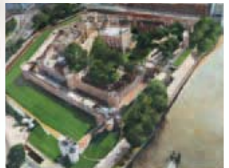
Today's Tower has many more buildings, including offices and barracks, but others, such as the Great Hall, have gone.
